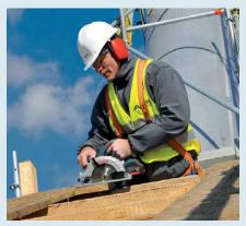
The cordless circular saw enables the user to have mobile use where safe to do so in places where it would otherwise be impractical.
