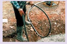
Robust, petrol powered machine, for the effective removal of air from wet concrete. Durable protection frame keeps machine safe in arduous site conditions.
