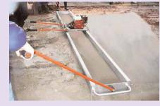
A twin vibrating beam screed for striking off and vibrating concrete between form work.
