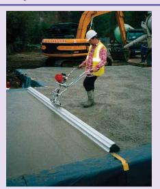
The Easy Screed has an easily detachable twin handle power unit that clamps on to beams of various lengths. The aluminium beam has a profile suitable for 'free screeding' or by reversing the same beam can be used for striking off across from formwork.
