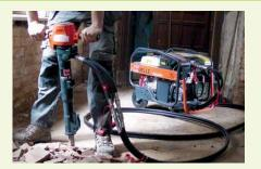
This hydraulic power pack is a portable high performance alternative to the compressor. It will fit into a small van and is ideal for breaking roads, paths, patios and drives.
