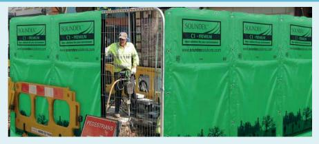
Designed specifically to provide high-absorption acoustic screening around site plant and other high noise emitting activities, their unique Velcro fastening ensures a seamless noise barrier with eyelets on all edges to enable easy suspension.
