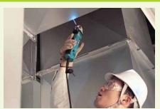
A compact drill with a fixed 90 degree head to allow access to awkward areas.
